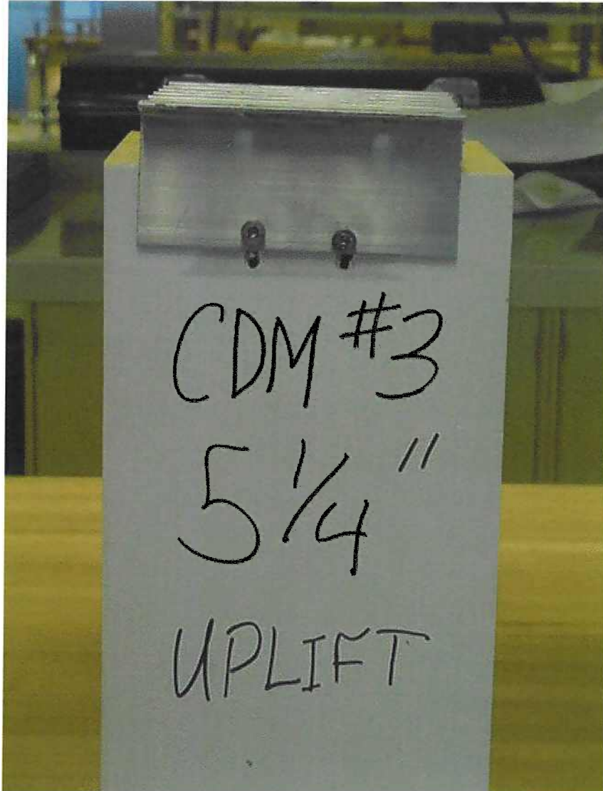
Photo No. 8 5-1/4" by 5-1/4" Porch Post Screw/Porch Post Failure
