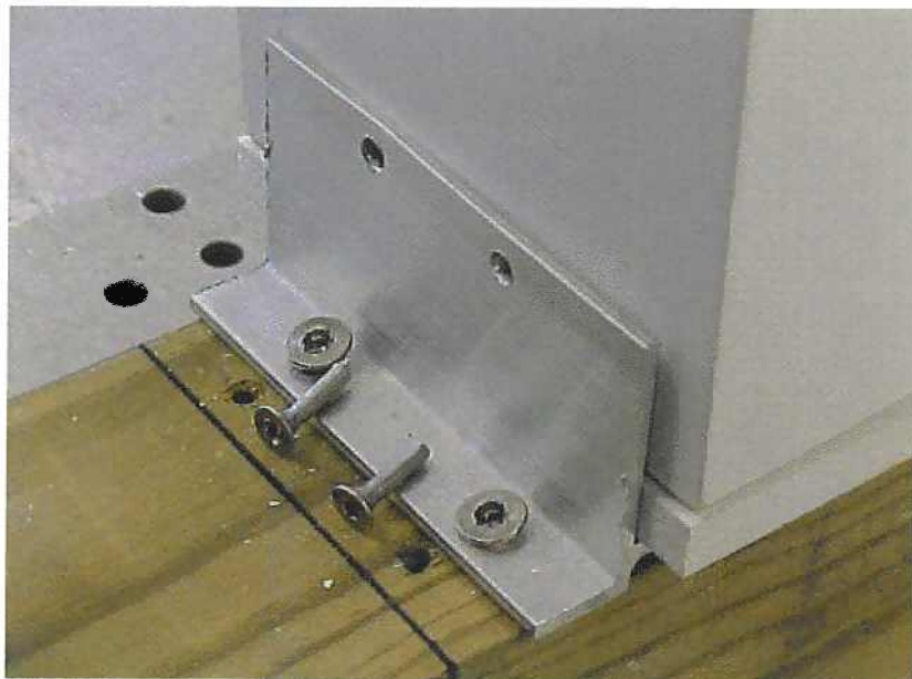
Photo No. 9 4-1/2" by 4-1/2" Porch Post Shear Failure of Screws
