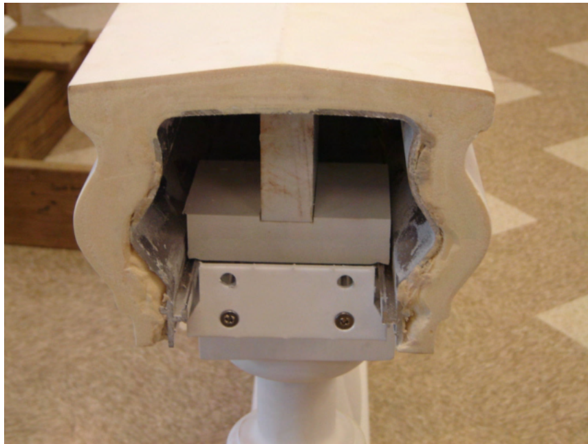
Photo No. 4 Top Rail w/Bracket
