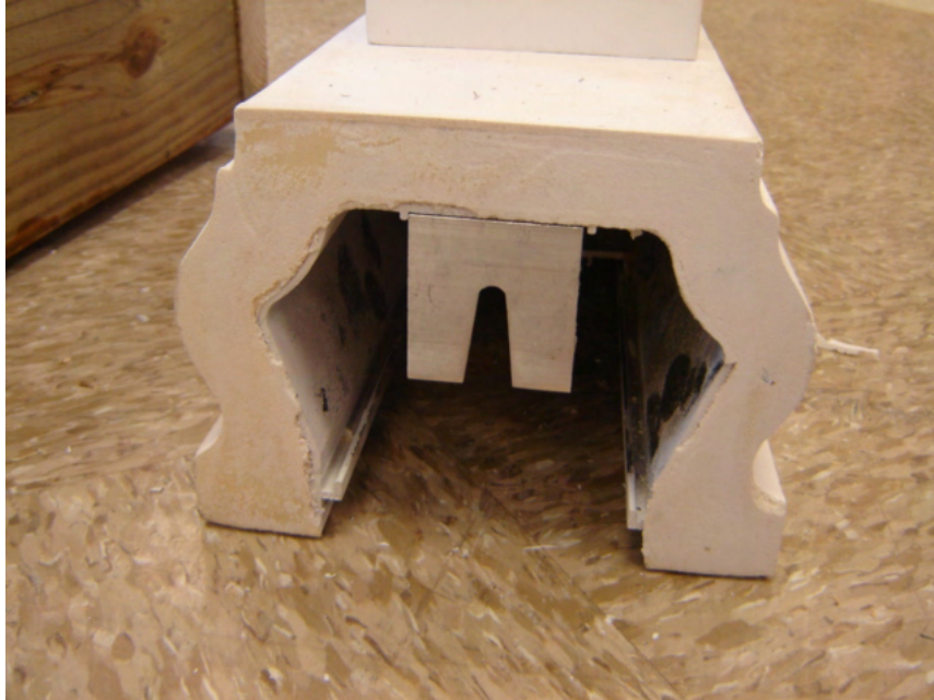
Photo No. 5 Bottom Rail with Bracket
