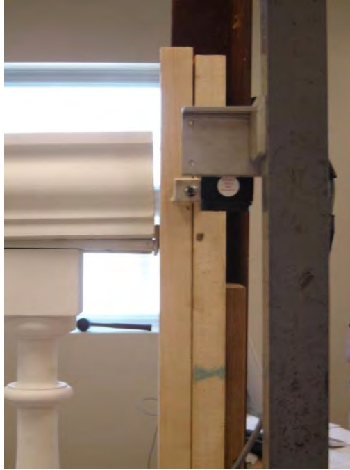
Photo No. 3 Top Rail Bracket Attachment into Wood Supports
