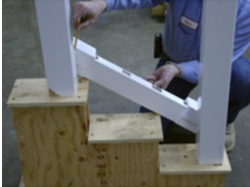
ends. Tape brackets so they won't slide on the rail. Cut carefully on scribed lines. Put rail back into place. Raise to proper position and secure to post, being sure screws are long enough to fasten into solid material.
