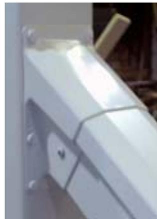
**ANGLED DECK INSTALLATION WITH ADJUSTA-BRACKETS:** With length calculated and brackets installed, simply use spacers (Cut off end pieces of 2 x 3 ½" Rail make good spacers) under rail to hold it level and the proper distance off floor and fasten screws to post.
